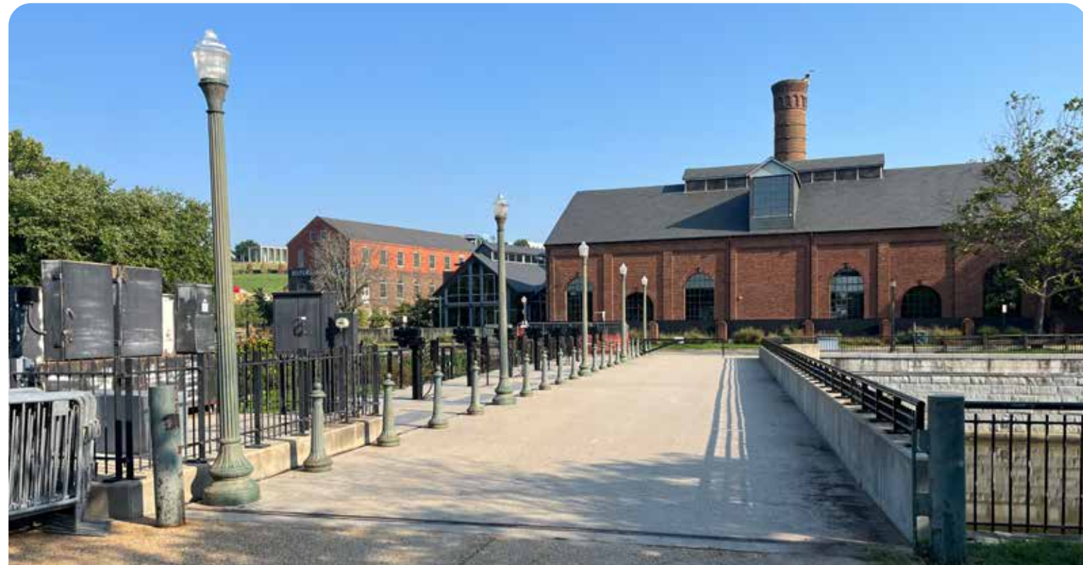
HAXALL BRIDGE LOOKING TOWARDS TREDEGAR
